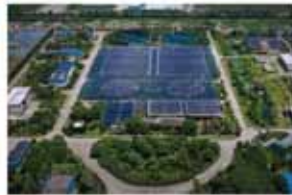
Sewage Water Treatment Plant Taizhou, Zhejiang, China 0.78MW 2015
