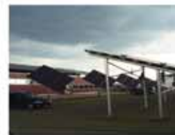
Bremen, Germany 180Kw 2011
