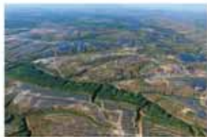
Eco-agri Solar Farm Datong, Shanxi, China 100MW Jun 2016
